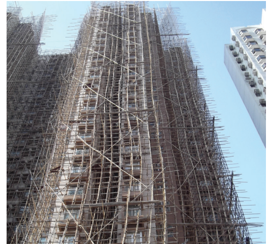
Figure 21: Bamboo scaffolding
